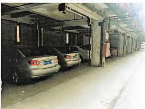
B区2层商铺现状-2
