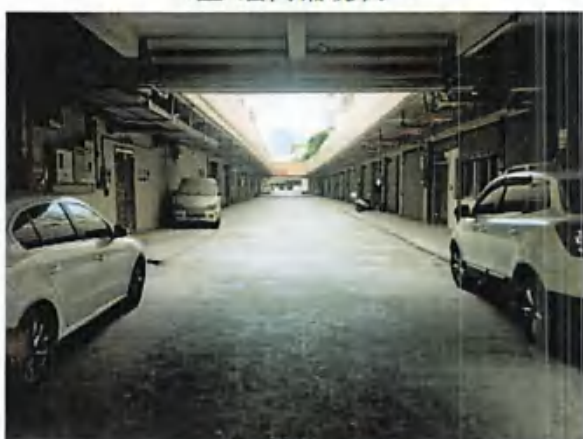
B区2层商铺现状-3
