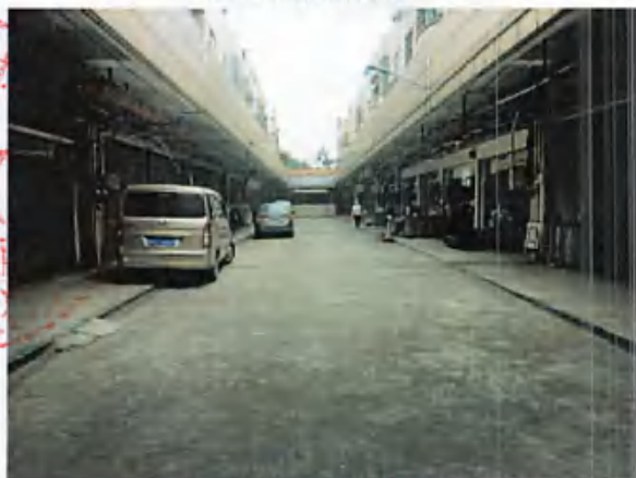
B区2层商铺现状-1
